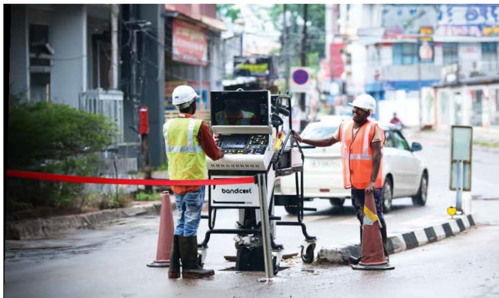
Figure 18: Robotic cleaning system for sewers (Bandicoot) (Genrobotics)
